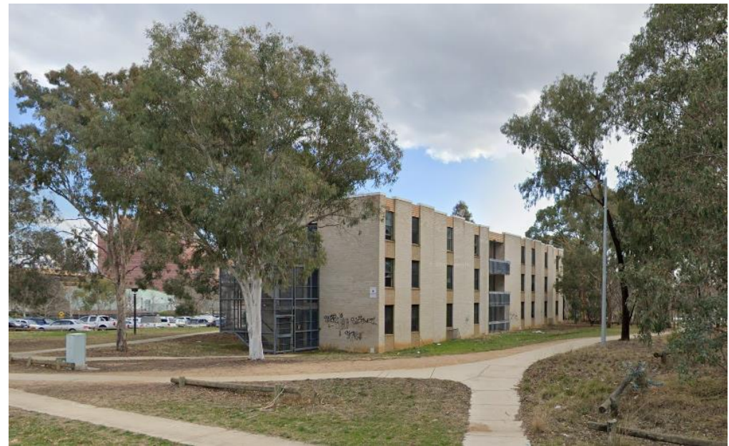
The building ceased student housing functions and fell into dilapidation in the 2010s, being demolished in 2020.
